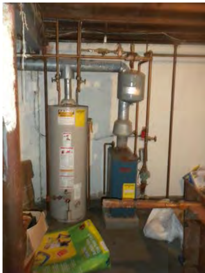
Typical boiler and domestic hot water systems
