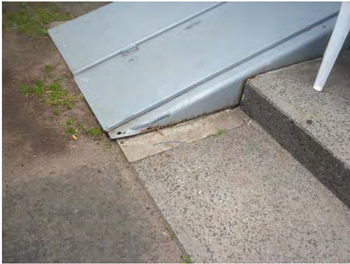
Rusted bulkheads set at ground level are causing water infiltration
