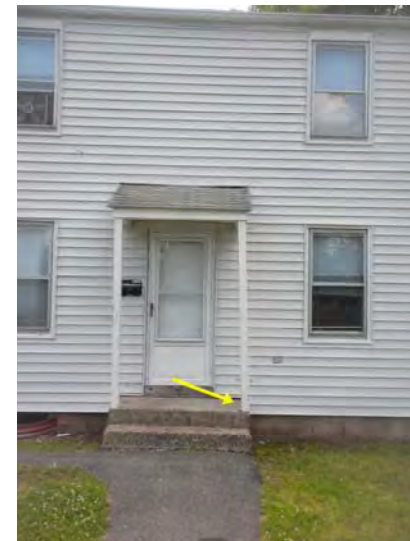
Deteriorating canopy and leaning canopy post
