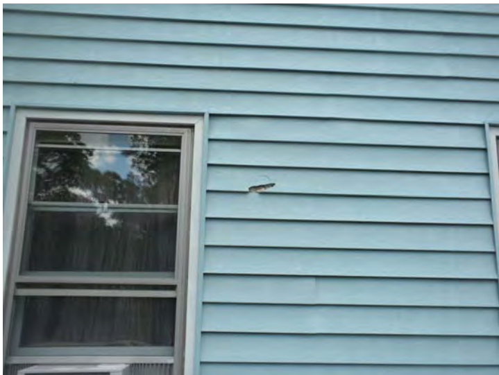
Cracked vinyl siding
